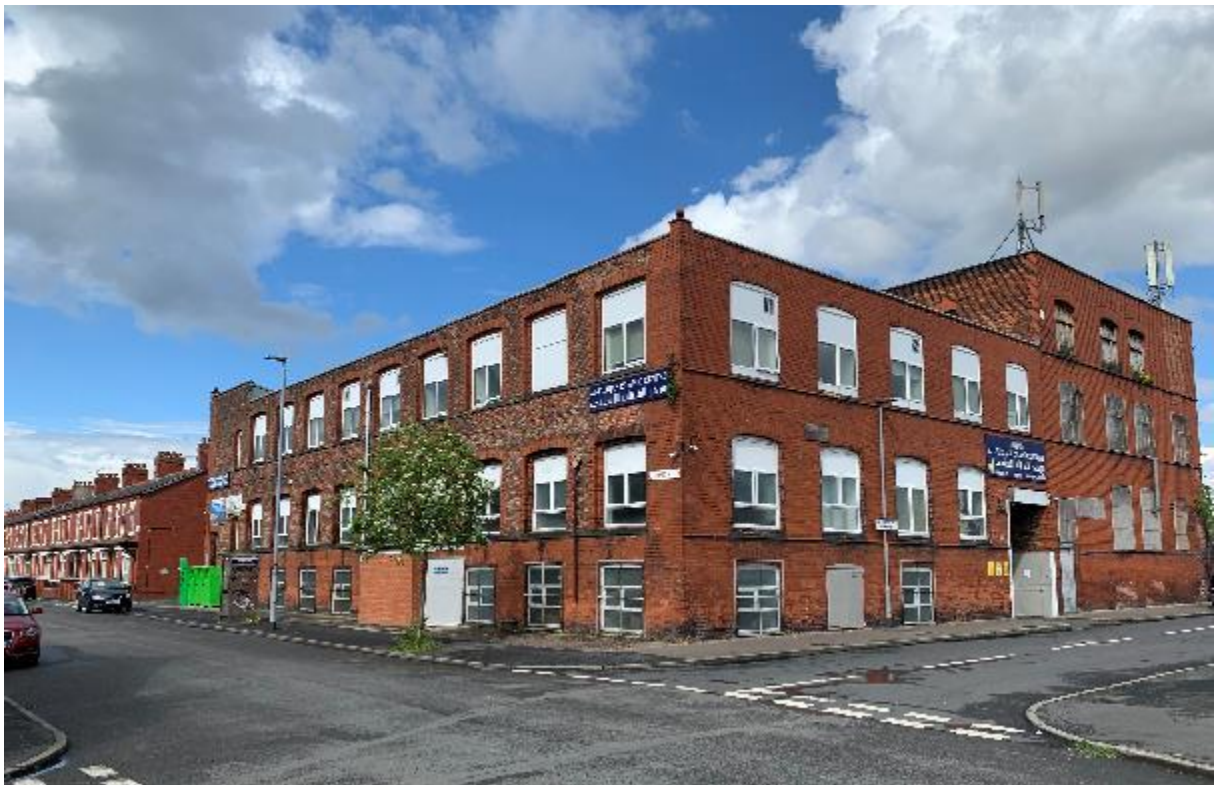
Photograph 2 View of the site looking North West from the corner of Crofton Street and Great Western Street
